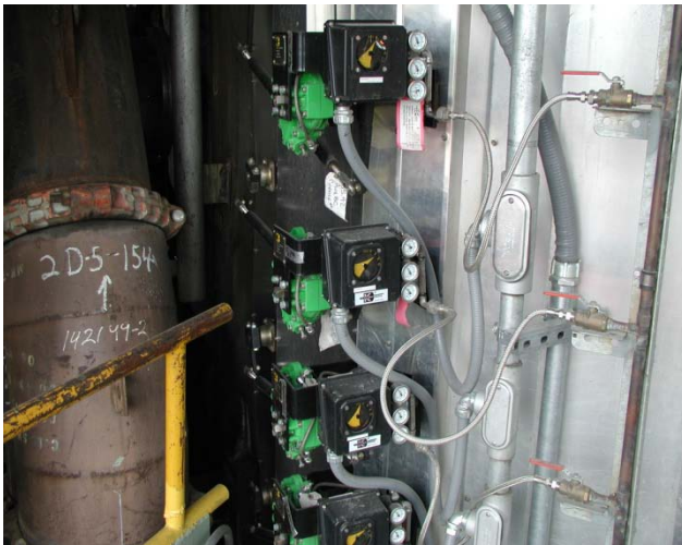
Fig. 3 Type K Windbox Drives in tight spaces
